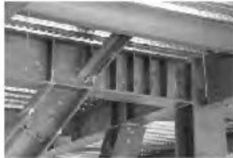
Typical initial course of Structural Engineers, Inc.
